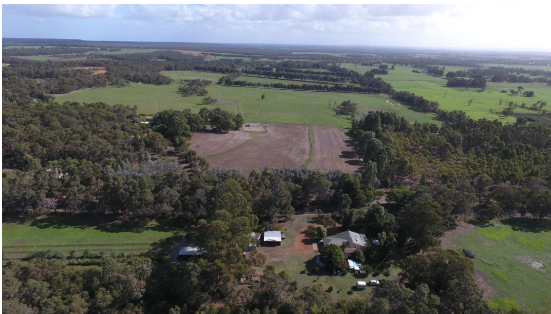
Figure 2. Location of Busselton agricultural property, site of first CellCube battery installation in WA.
