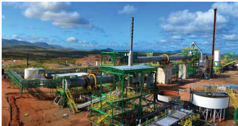
A view of the vanadium operation at Maracás in Brazil, controlled by Largo Resources.
