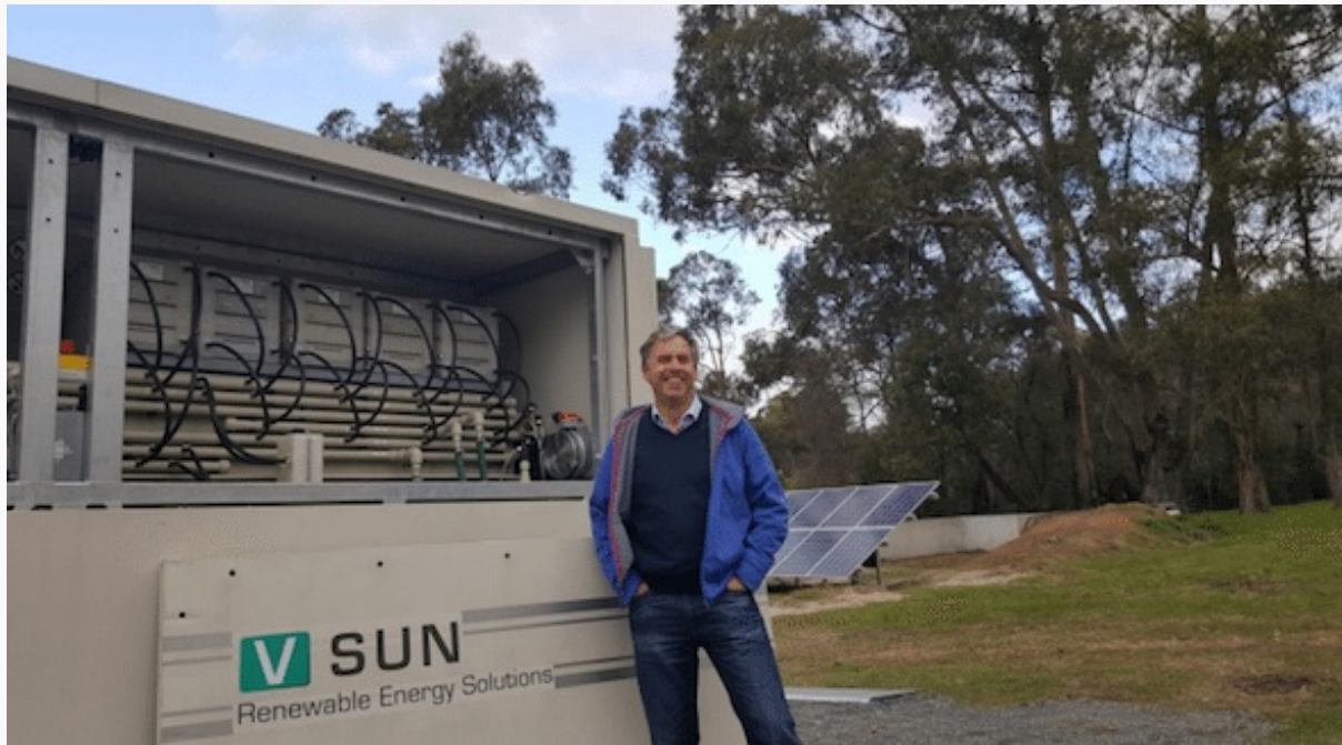
AVL managing director, Vincent Algar, next to the CellCube vanadium redox flow battery.
